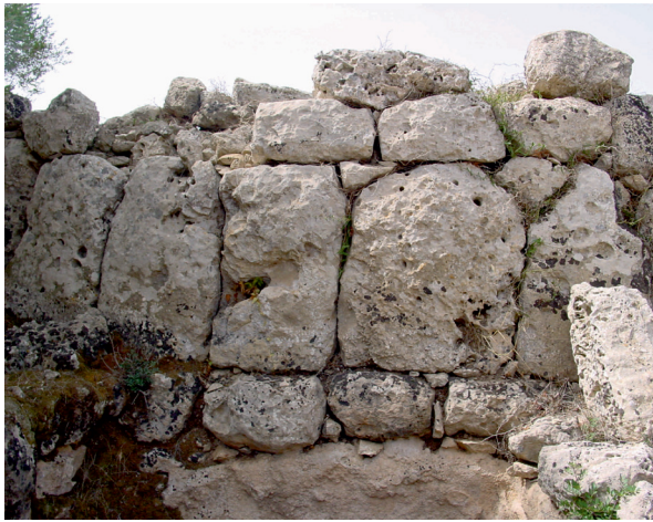
FIG. 4. Example of the monumental rigging in Circle 2 of Sant Vicenç d'Alcaidús (Menorca) (photograph provided by J. de Nicolás).
