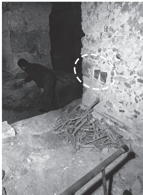
FIG. 8. Church of Sant'Eufisio, Nora. Detail of the restoration and research works conducted in 1977. The location of the inscribed stele is indicated by the circle (with permission of the Soprintendenza A.B.A.P. per la città metropolitana di Cagliari e le provv. di Oristano e Sud Sardegna; photographic archive, n. 15275).
